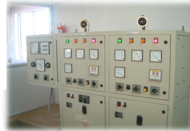
The power delivery panel
